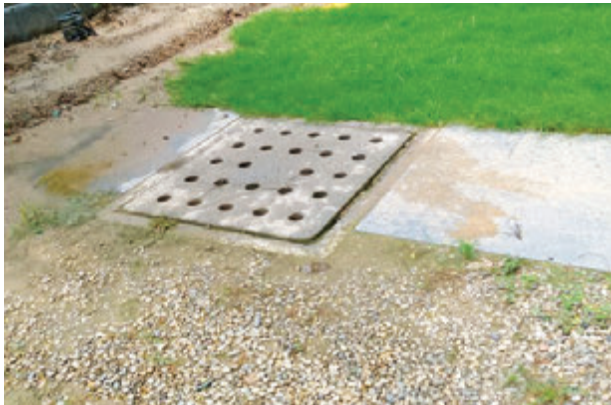
Storm water connection outside building premises
