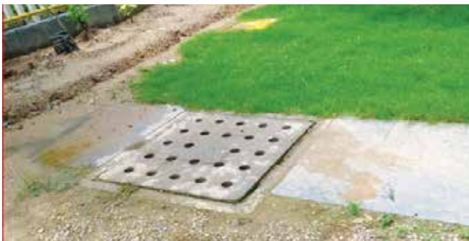
Storm water connection outside building premises
